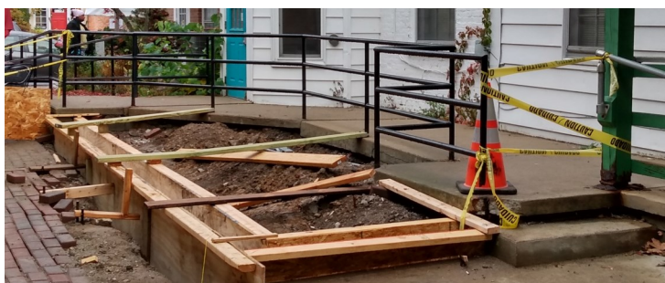
The new patio taking shape in October, 2022
